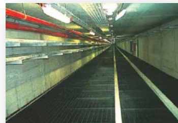
Tuas Undersea Cable Tunnel, Singapore (Completion:1998) GGBS ratio= 70%
