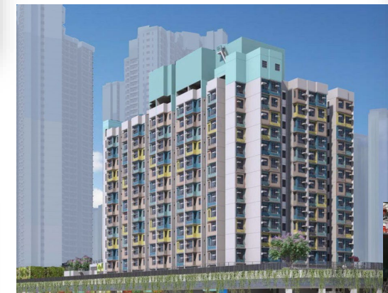
Public Housing Development at Tung Chung Area 99
